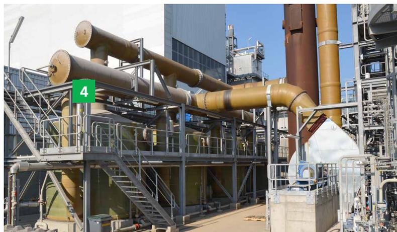
The final step of the gas cleaning process is the activated carbon filter, a series of four filters in parallel to remove the dioxins, furans (PCDD/F) and heavy metals (such as mercury) from the flue gases.
